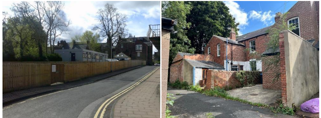
Fig 53 above. An image of the stark timber fencing along Territorial Lane, and the rear of Gladstone Villas where historic back yard walls have been removed impacting negatively.
