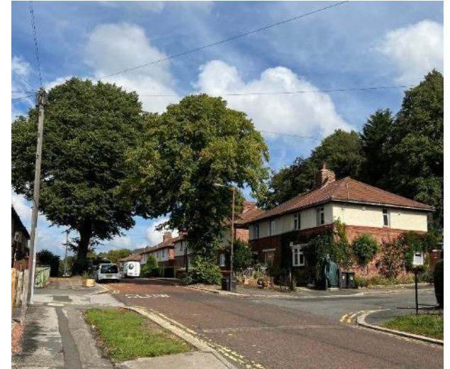
Fig 56 below. Images of typical street scenes within Whinney Hill, semi-detached and larger blocks of social housing, with some short cul-de-sacs enhanced by an abundance of greenery in the public realm.
