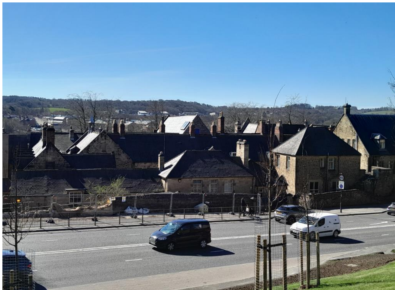
Fig 68 below. An image from Lower Gilesgate that captures the roofscape of The former College characterised by traditional slate roofs with ridged punctured by chimneys.
