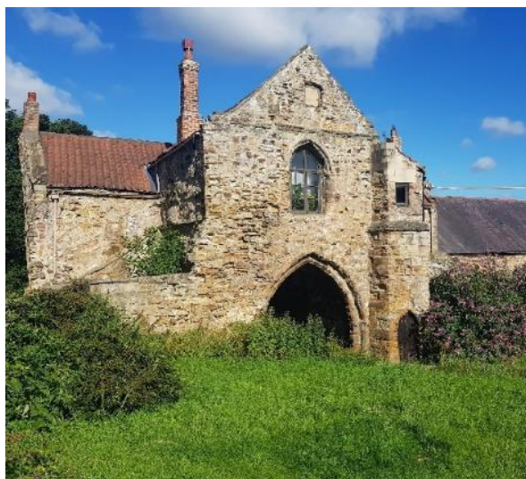
Fig 20 above. The grade I listed Kepier Gatehouse.
