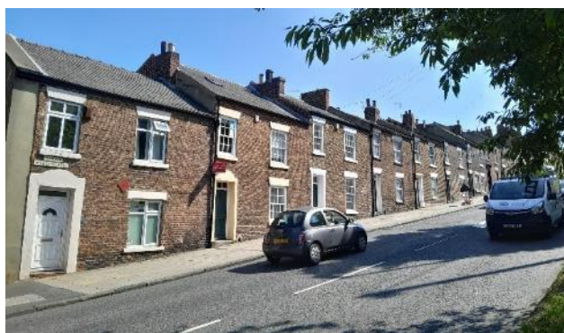
Fig 30 above. The short historic side street at Magdalene Street and the 19 th century properties lining the north side of Gilesgate Bank.
