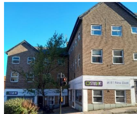
Fig 45 below. The buildings and sites identified as impacting negatively on the character and appearance of the area.
