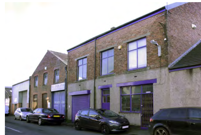
Peel Street industrial buildings
