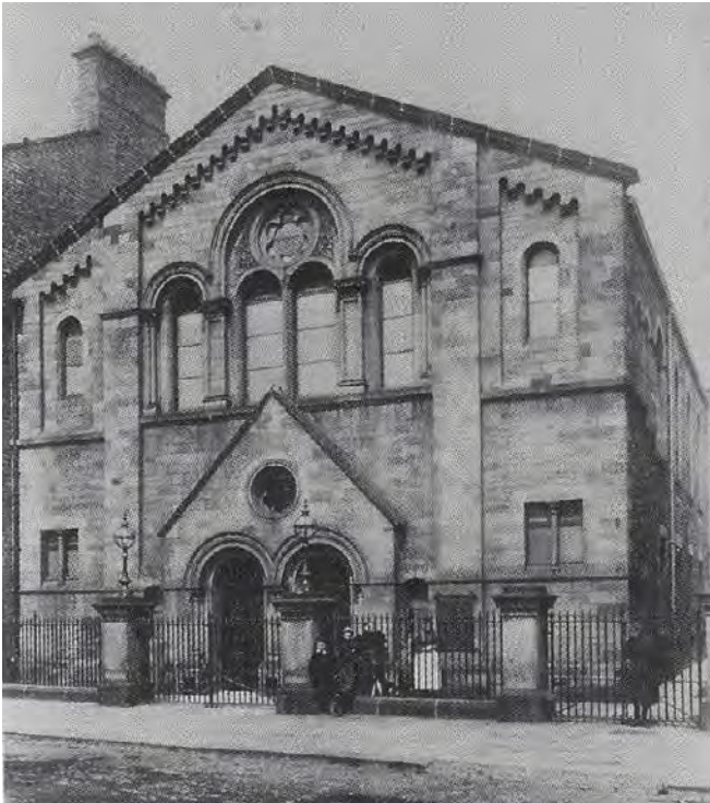
North Bondgate Wesleyan Chapel following rebuilding
