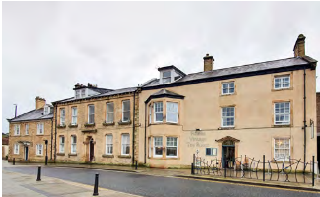
Many of the buildings around Market Place are listed; for example, Nos.9, 9A and 10 Market Place are all Grade II listed
