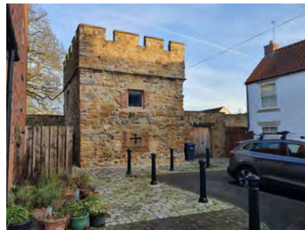
West Mural Tower marks a former entrance into the Castle complex
