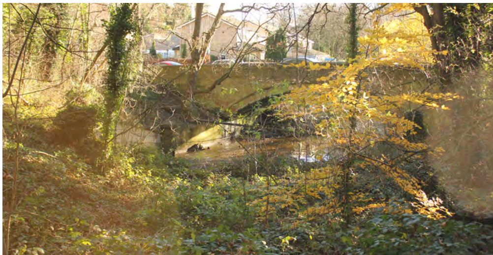
Bridge over the river Gaunless, Durham Chare
