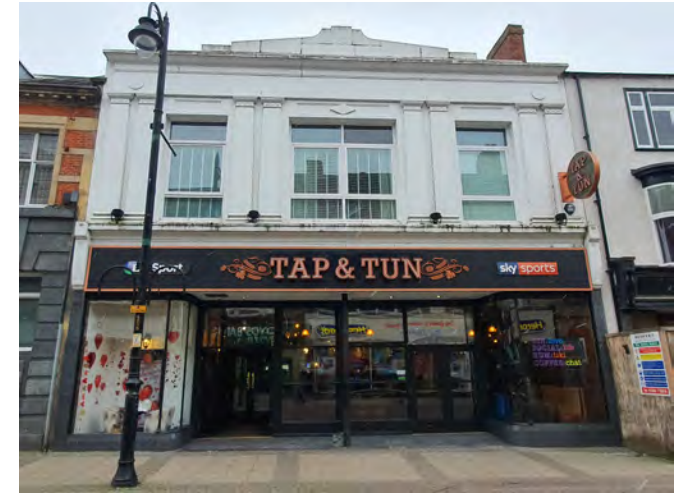
Art Deco former purpose-built Marks and Spencer
