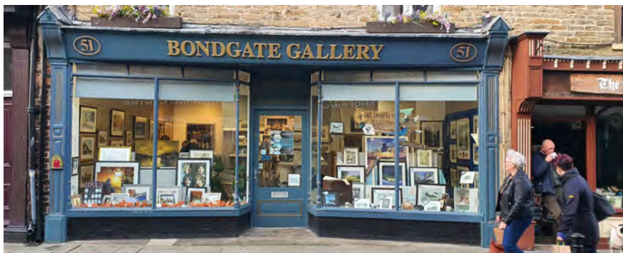
Traditional shopfronts in Fore Bondgate
