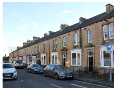
Grander terraces on Victoria Avenue
