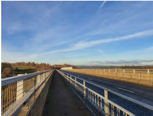
The Newton Cap Viaduct as converted for road traffic.
