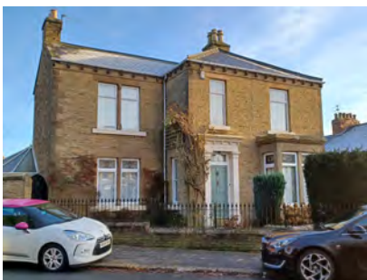
End-terrace villas on Etherley Lane
