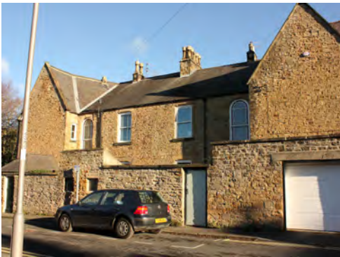
The back of villas on Park Street
