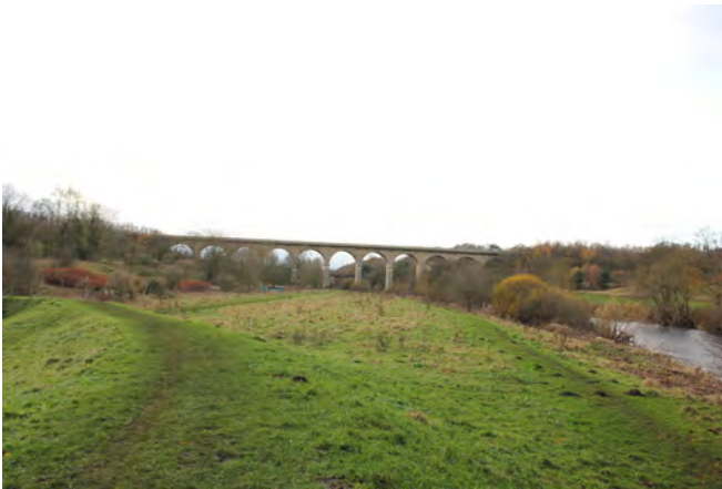
Riverside walk along the Wear, looking west at the Newton Cap Viaduct
