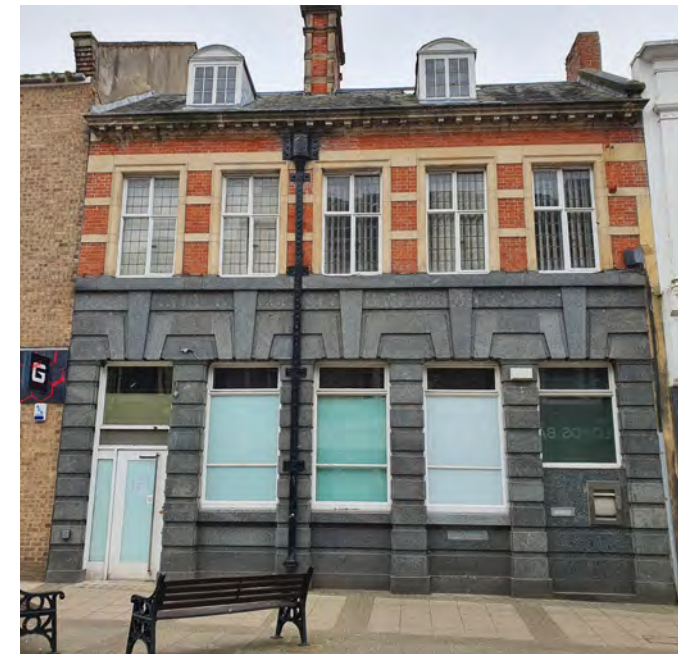
Unusual Georgian-style former bank on Newgate Street with rusticated granite ground floor
