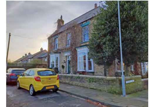
End of terrace villa, Clarence Street
