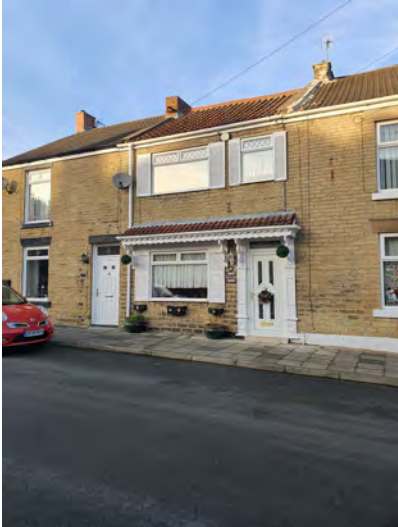
Loss of original windows and openings and a desire for individuality has made this house unrecognisable as a Victorian worker's cottage
