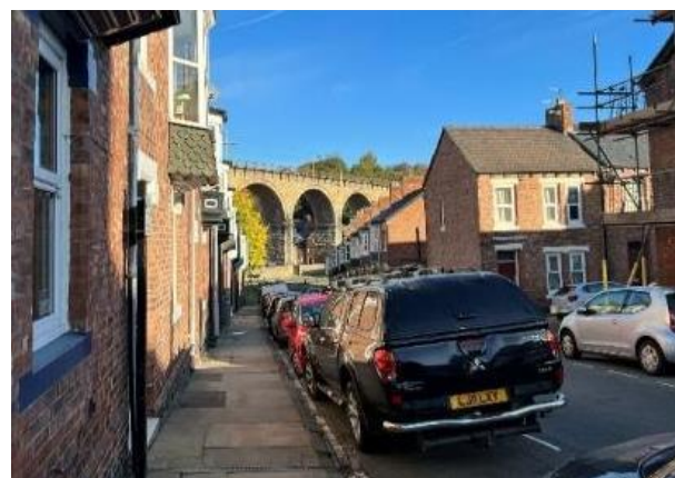
Fig 54 below. Examples of on-street parking cluttering historic residential streets.
