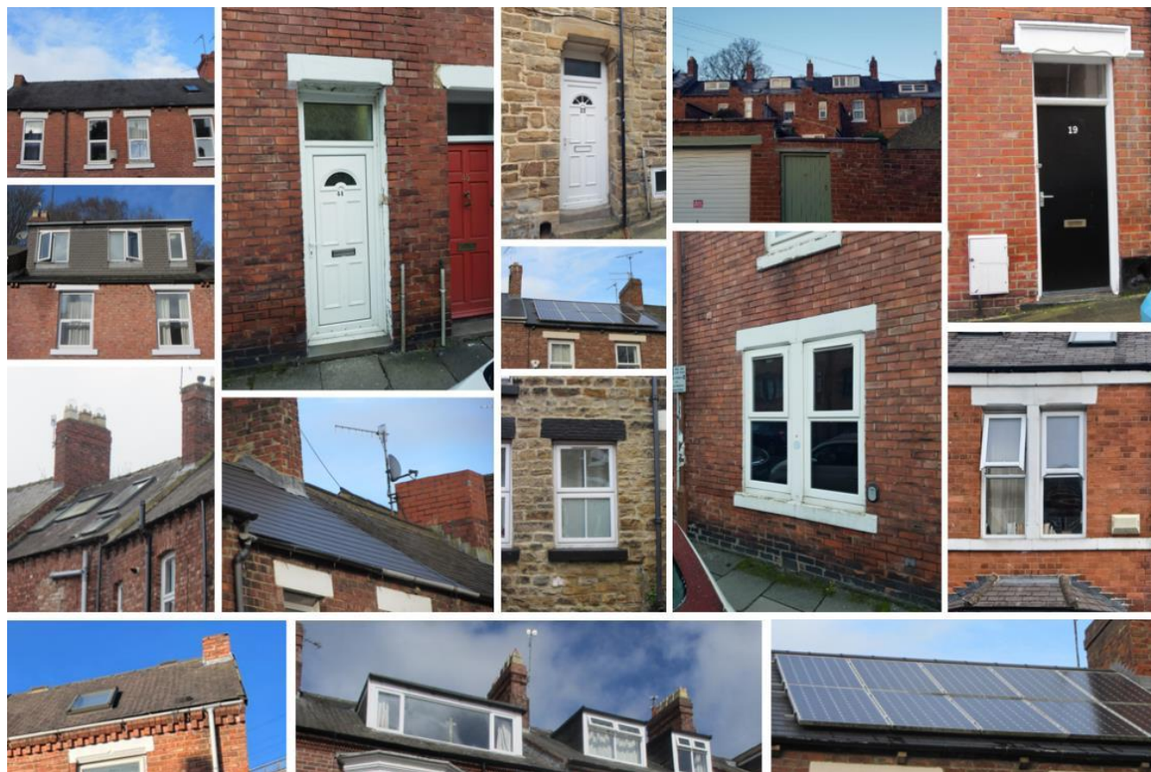
Fig 53 below. A selection of images showing examples of unsympathetic alterations to historic buildings within the character area.
