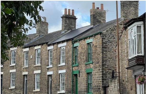
Fig 48 below. Colpitts Terrace, former Rington’s Tea workshop and Percy House.
