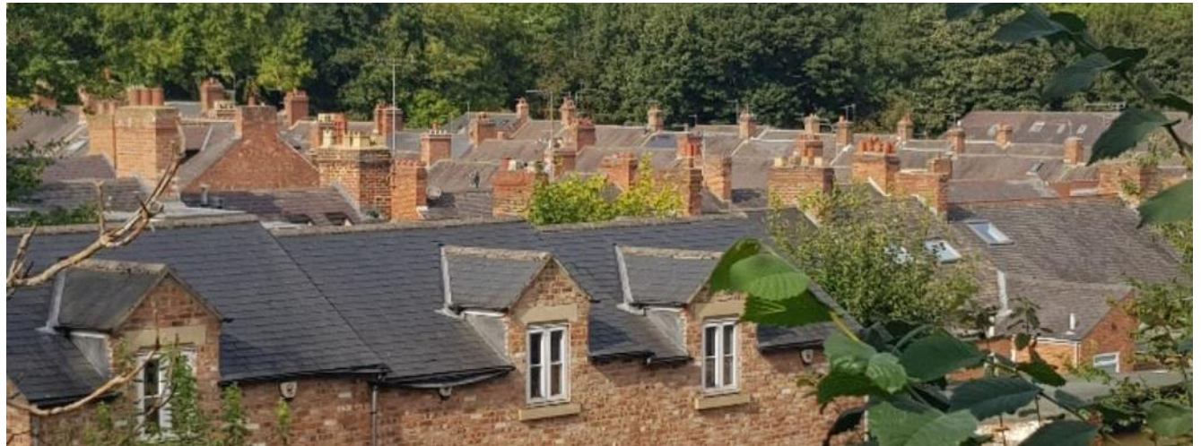
Fig 50 below. Images showing different roofscape across the Victorian terraces at Hawthorn Terrace, Palatine View, Crossgate Peth and Lawson Terrace.
