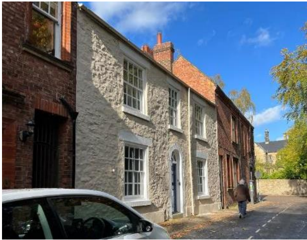
Fig 67 above The varied brick and rendered historic buildings fronting Pimlico.
