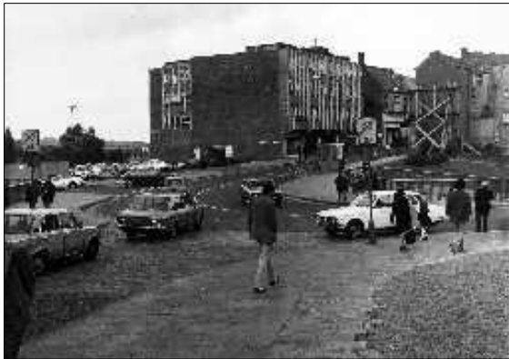
Fig 21 above. A view of lower Claypath in the 1970s, Durham County Records Office (Ref.DR00921), now the site of the Walkergate Development.
