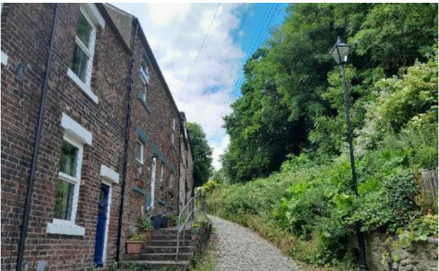
Fig 88 below Sidegate, Albert Street and Redhills Miners Hall.
