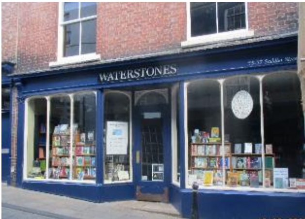
Fig 61 below. Examples of different shop fronts good quality traditional designs and lower quality modern designs with poor signage
