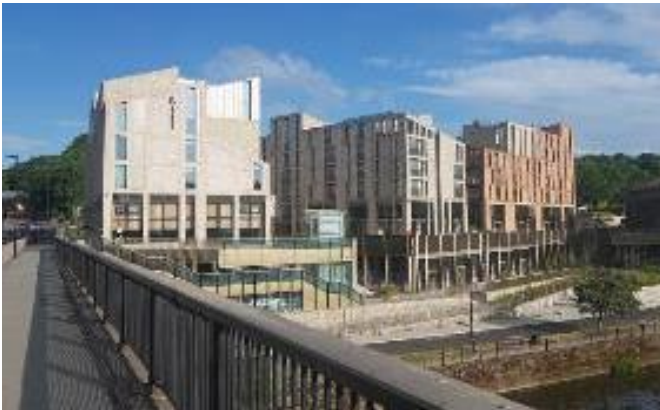
Fig 53 above. A view of the contemporary mixed use riverside development at Milburngate taken from Milburngate Road Bridge.
