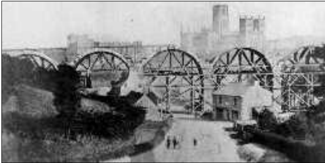
Fig 15 above. The construction of Durham Railway Viaduct 1857, © County Records Office.
