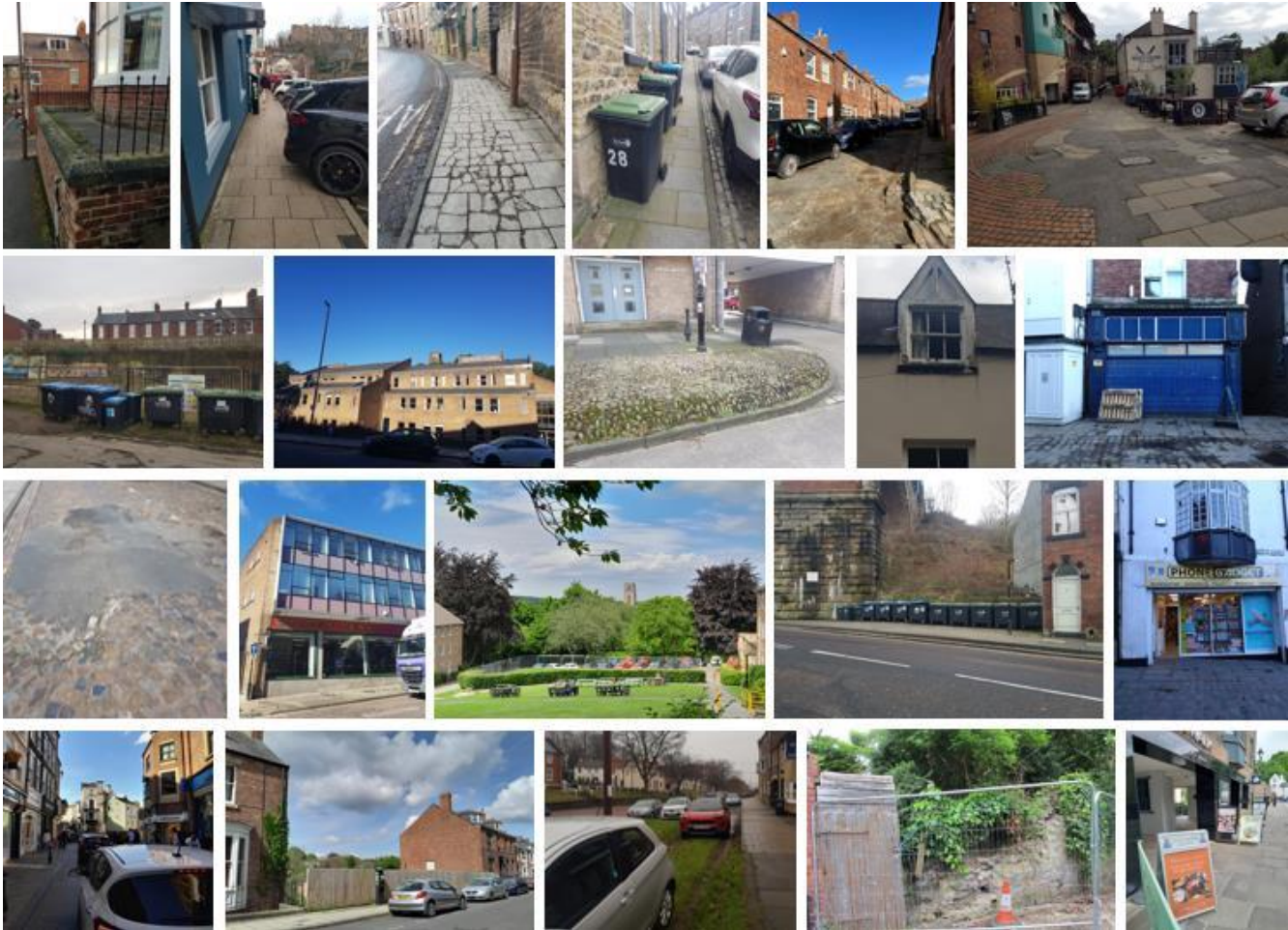
Fig 60 below. Examples of the issue and problems found within the conservation areas.
