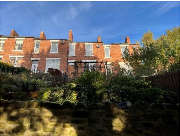
Fig 79 above. Diamond Terrace, the terraces displaying typical period characteristics despite unsympathetic modern alterations.
