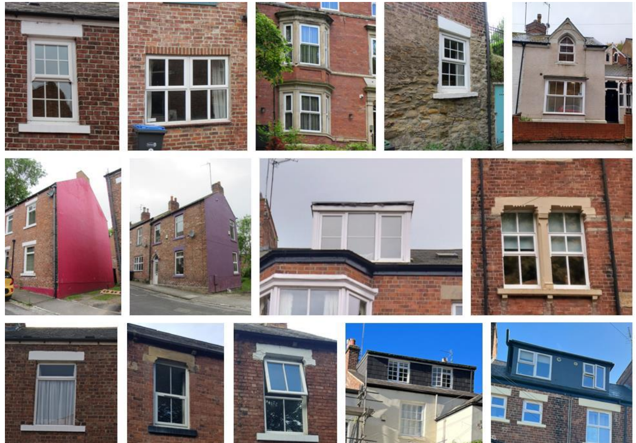
Fig 52 below. A selection of images showing some of the negative alterations to historic buildings within the character area including imitation sash uPVC windows, painting historic brickwork, and large flat roofed dormers.
