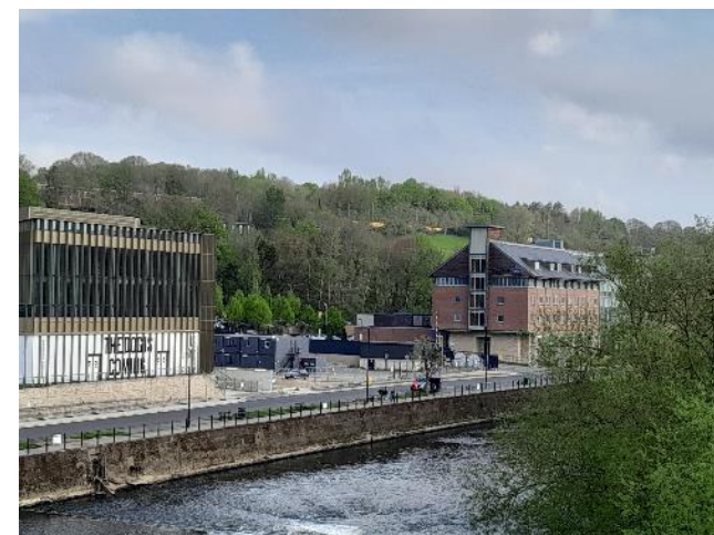
Fig 96 below. A selection of images showing the negative issues and problems identified, gap side at the riverside, poor degraded surfacing, and empty retail units.
