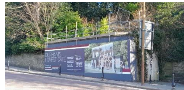
Fig 51 below. The boarded over former public convenience at North Road.
