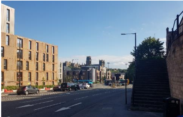
Fig 36 above. Images showing the contrast between the north and south parts of Framwellgate Peth, an open layout enhanced by greenery that becomes an enclosed route dominated by large scaled modern developments.
