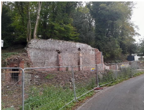
Fig 49 below. The site of the cleared historic industrial buildings.
