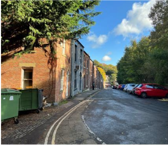
Fig 38 below. A series of images of the general street pattern and character of different routes within the character are. Below left: Redhills Lane and Obelisk Lane. Middle: Station Approach. Right Fieldhouse Terrace and Princes Street.
