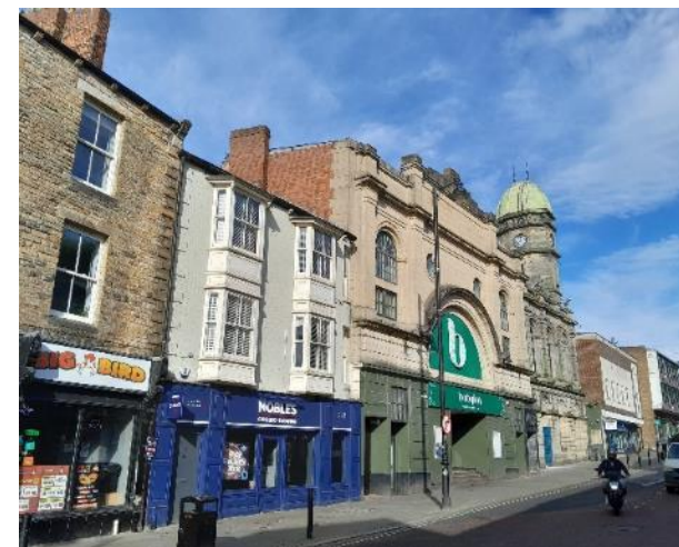
Fig 67 below. Views within North Road with the former cinema and miner's hall focal points, and the distinct contrast between the 19 th century Methodist Minister's House and contemporary bus station redevelopment.
