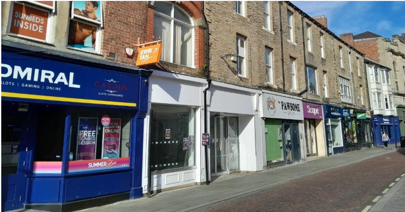
Fig 74 below. The commercial street scene on the south side of the street showing the wide range of different shop fronts and signs on display.
