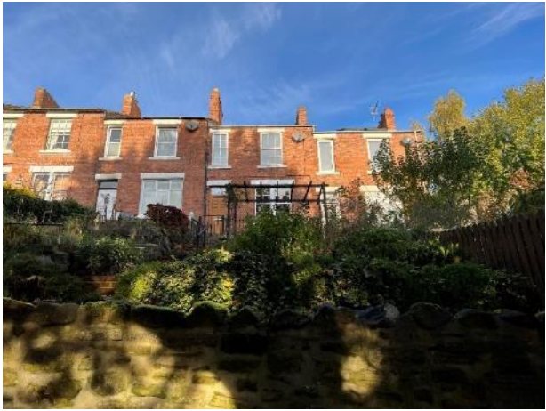
Fig 82 above. Diamond Terrace, the terraces displaying typical period characteristics despite unsympathetic modern alterations.
