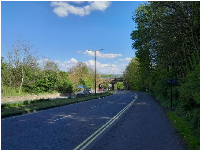
Fig 53 above. The north end of Framwellgate Peth travelling into the city with a positive green character.
