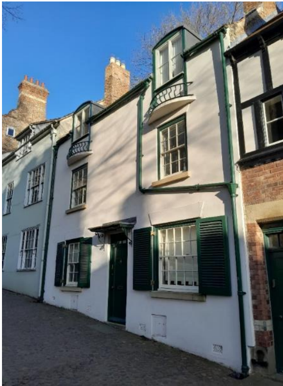
Fig 22 below. Dun Cow Cottage, while externally it appears to be 18 th century it is probable that it includes earlier possibly medieval fabric, and the tradition is that this site is that of the bishops' stables. Right: No 5 Owengate of the late medieval period and one of the few buildings in the city where the timber-framed construction is visible.
