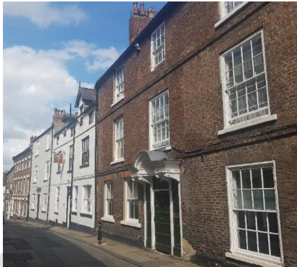
Fig 61 below. Views along North and South Bailey showing the Durham Vernacular style.
