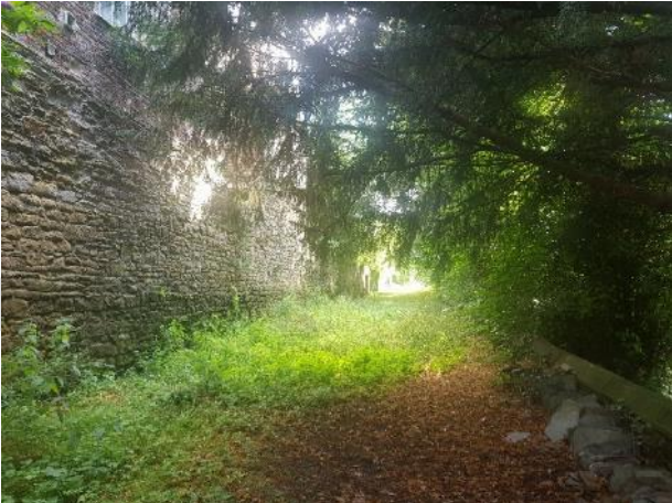
Fig 77 below. "Prebends Walk, an early feature of c.1680 that provides space for recreation outside the city walls and a place from which to view the river, and a typical stepped route through the woodland.
