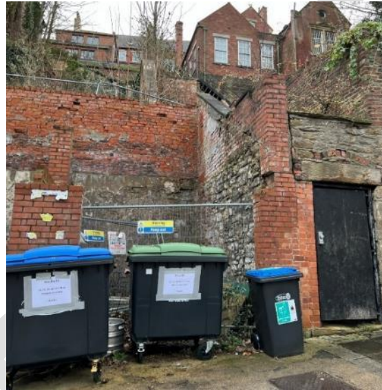
Fig 46 below. Examples of the negative elements identified, the disused site at Back Silver Street, Nos 17-18 Market Place “Tesco”, the riverside elevation of Prince Bishops Shopping Centre, and poor security shutter to a long term vacant retail unit.
