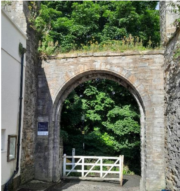
Fig 19 above. The Water Gate at South Bailey, a scheduled monument.
