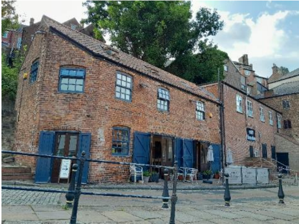
Fig 43 below. The unique riverside industrial buildings at Fowlers Yard.
