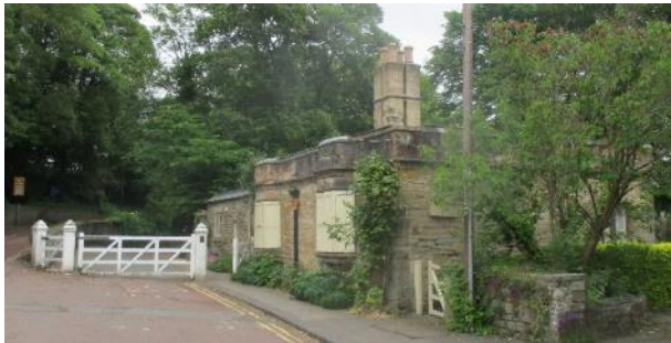
Fig 79 below. Prebends Gate Lodge and Cottage.
