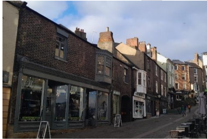
Fig 45 below. Images of general roofscape views at Elvet Bridge, Silver Street, and the Market Place showing the differences in roof pitches, ridge, and eaves levels, with rooflines punctured by gables and chimneys.
