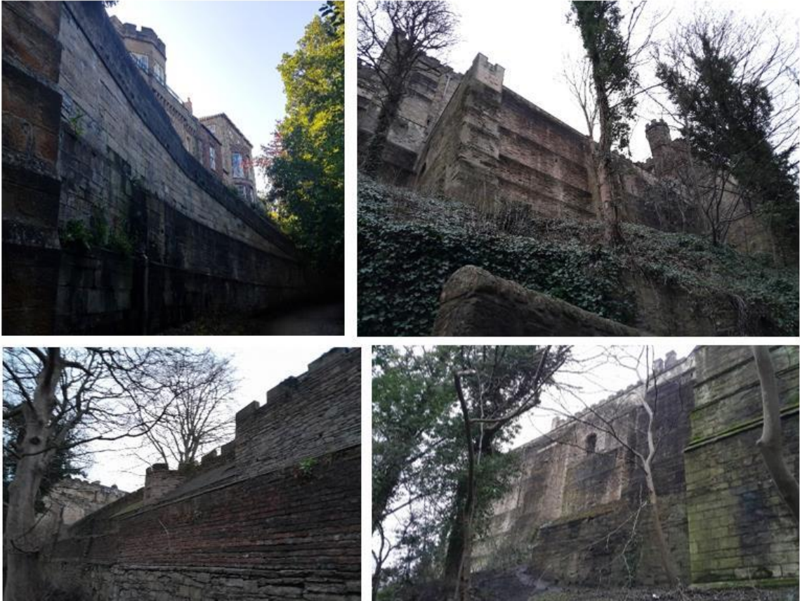
Fig 68 below. A select of images showing different sections of the city defensive walls and terraced walls around the riverbanks, showing separate phases of construction and large buttress features.
