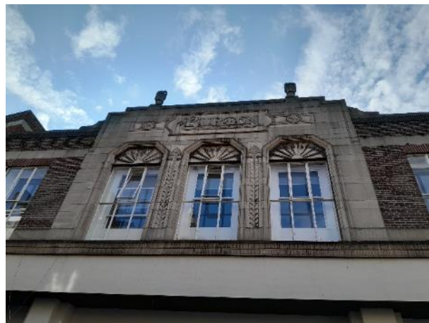
Fig 40 above. The distinctive Art-deco upper floor of Nos 7-8 Silver Street.
