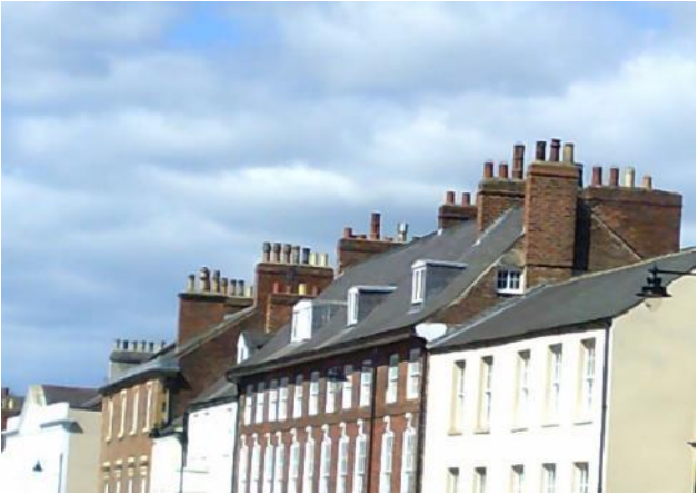
Fig 47 below. A close up view of the roofscape along part of Old Elvet with positive interjections in the form of landmarks such as the church spires and copper dome of Hotel Indigo, formerly Old Shire Hall.
