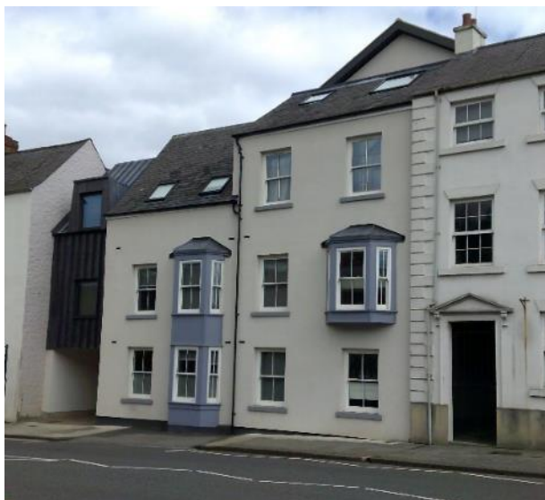
Fig 46 below. The contemporary infill development at the former Three Tunns Hotel successfully completing the streetscene and an extension at 31-33 Church Street.
