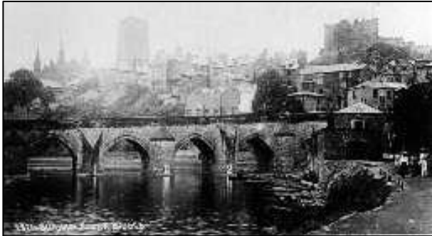
Fig 17 above. View of Elvet Bridge from original postcard c.1910 Durham County Records Office (Ref.DR00747),
