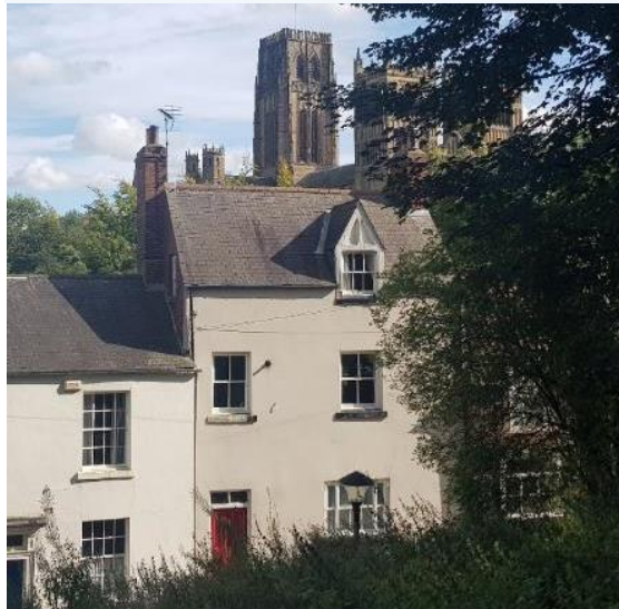
Fig 8 above. The view of the cathedral towers above the buildings on South Street taken from St Margaret's graveyard.
