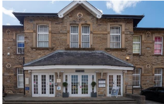
Fig 32 below. A selection of images showing the variation in building ages, forms, and styles within the area.
