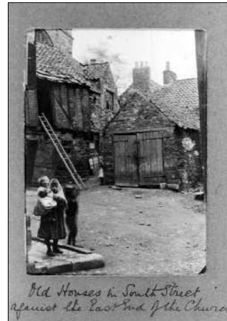
Fig 14 above. Old houses in South Street against the east end of the church South Street 1901-1925 Durham County Records Office (Ref.DR01017).
