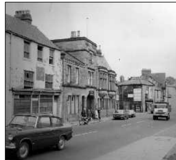
Fig 13 above. The bottom of Gilesgate Bank the Durham Ox public house and DLI Drill Hall demolished to make way for the new through road c.1961-67 Durham County Records Office (Ref.DR00949),
