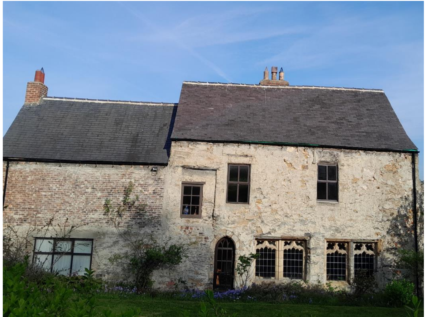
Fig 79 below. The rear of the farmhouse is particularly notable being of a rubble construction with partial boulder plinth, and including an ogee-headed entrance door, windows with Perpendicular tracery and irregular windows including a blocked opening.
