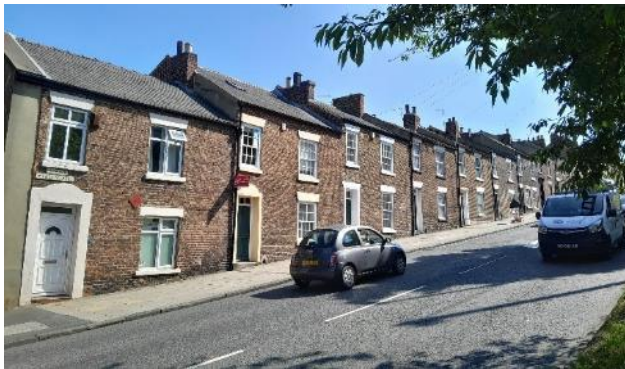
Fig 29 above. The short historic side street at Magdalene Street and the 19 th century properties lining the north side of Gilesgate Bank.
