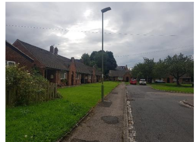
Fig 31 above. McNally Place a characterful small housing area of bungalows grouped in pairs around an open central space.
