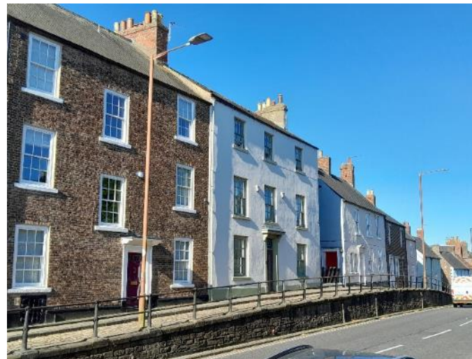
Fig 38 below and right. A selection of images showing different architectural styles and character that define the character area.
