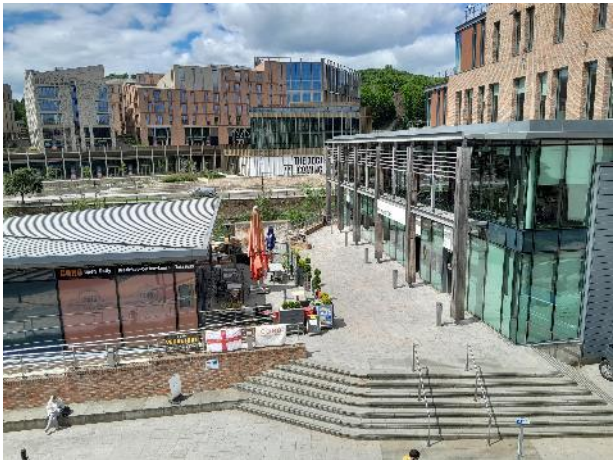
Fig 86 below. A selection of images of the contemporary public realm of different terraced levels, riverside walkway, and open urban square.
