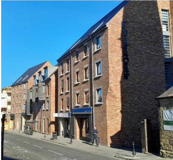
Fig 42 below. Positive modern developments within the character area the Army Reserve Centre, Student Castle, Claypath, and bungalows at McNally Place.
