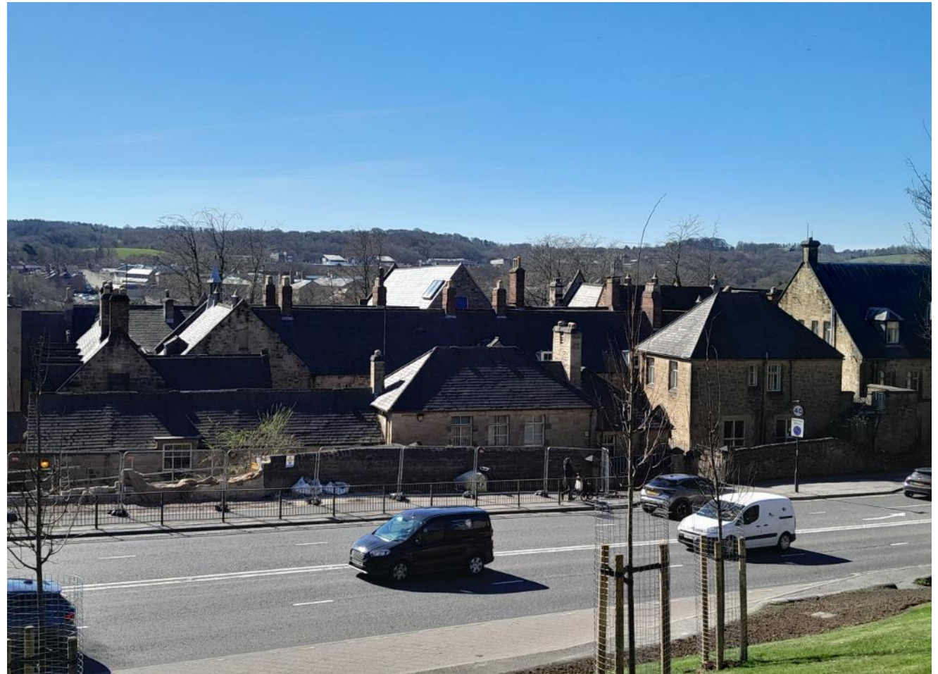
Fig 68 below. An image from Lower Gilesgate that captures the roofscape of the college characterised by traditional slate roofs with ridged punctured by chimneys.
