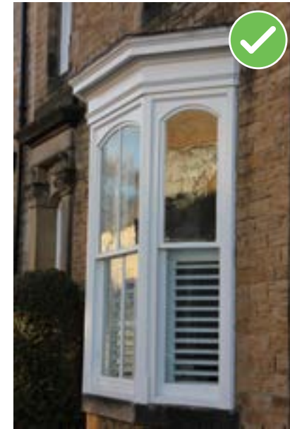
Traditional bay window in timber with lead roof
