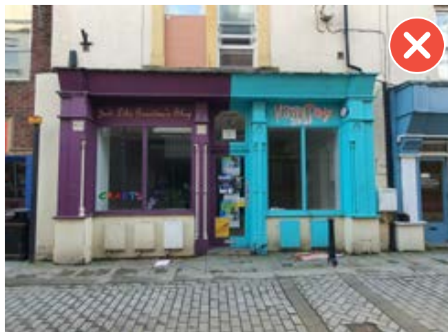
This paint colours of this traditional shopfront are garish and individualistic; future tenants should consider a more sensitive approach by choosing a single, muted colour.
