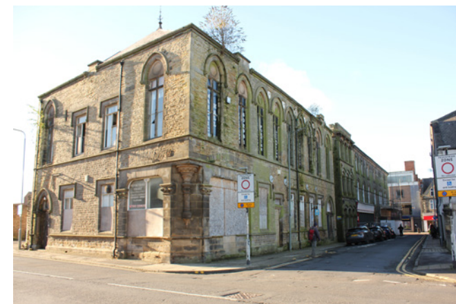
The vacancy of the Masonic Hall and the adjacent Mechanics Institute are severely impacting the appearance of the surrounding conservation area
