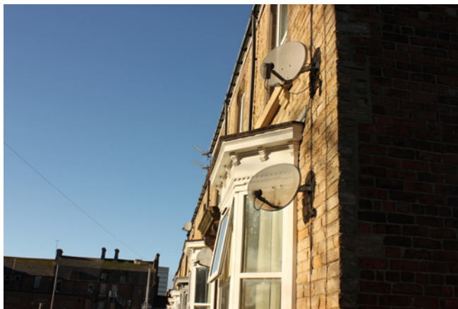
Satellite dishes and aerials proliferate on this terrace
