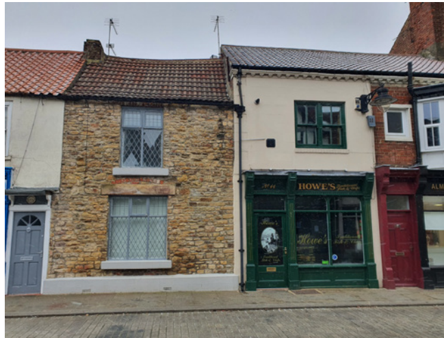
Mixed uses in Fore Bondgate
