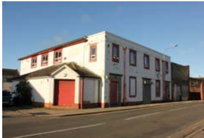
A mid-twentieth century building on Kingsway in poor condition
