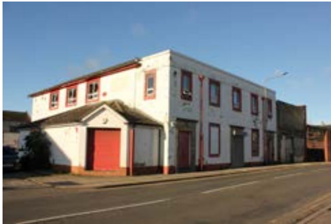
Detracting building on Kingsway
