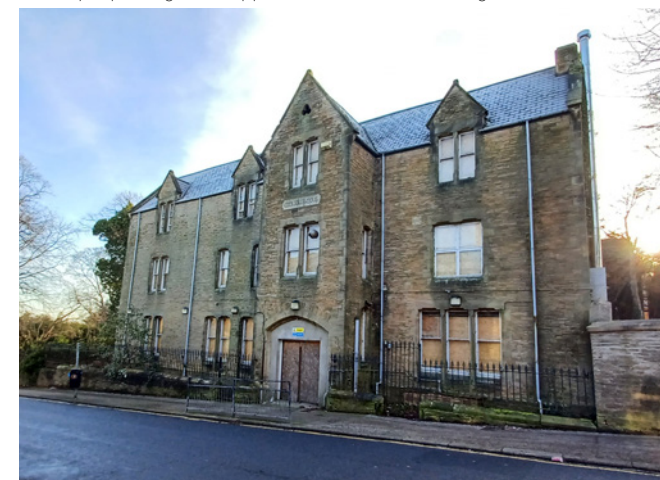
Clairmont, a vacant former maternity unit on Princes Street
