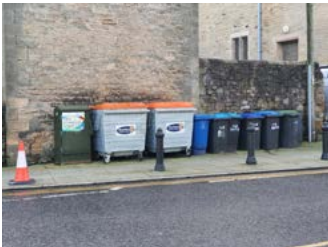
Commercial and domestic bins can negatively impact on the appearance of the conservation as here in Market Place
