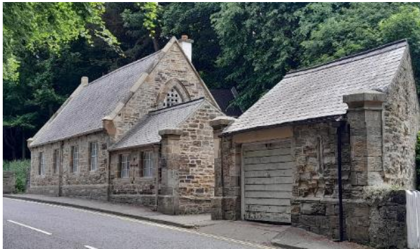
Fig 30 above. The 19 th century former coach house.
