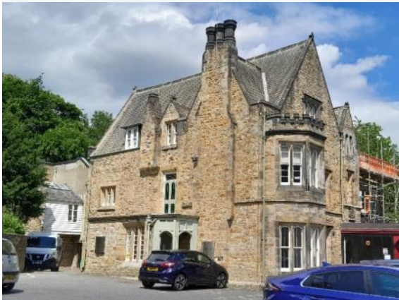
Fig 5 above. A 19 th century former private house.
