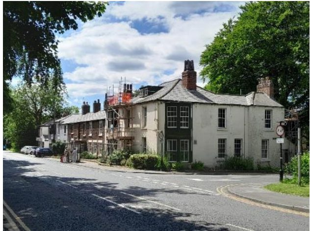
Fig 1 below. The conservation area has an interesting and distinctive mixture of historic buildings of different use and 20 th century purpose-built college buildings with their own distinctive architectural style.
