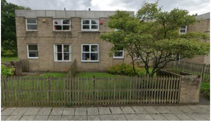
Fig 70 below. The low quality later accommodation and detached garage blocks.
