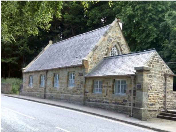
Fig 12 above. The grade II listed former coach house, saddle room, byre, hay loft and hen house of c.1868 recently restored.
