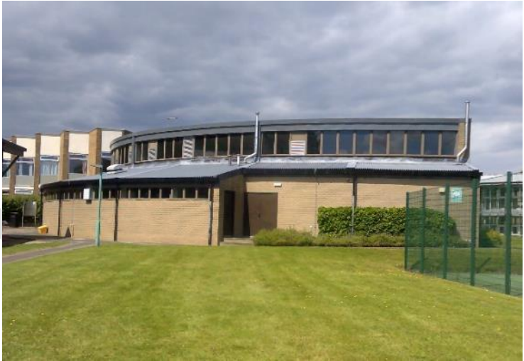
Fig 37 left and above. A later addition to the original east wing and above the Lindisfarne Centre on the site of what was originally supposed to be a chapel building.
